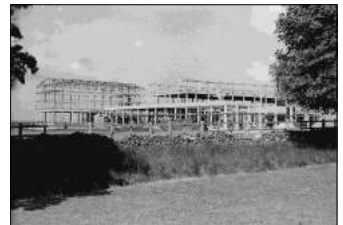
Manor School under construction, 1962
