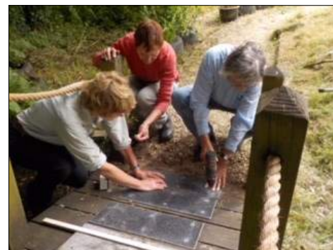
Attaching a non-slip surface to a bridge
