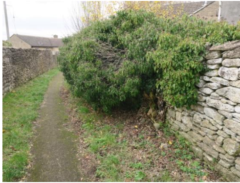
Top heavy and in danger of collapse
