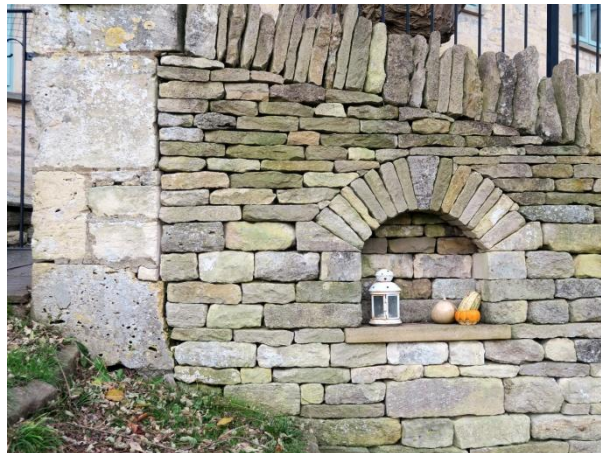
New 'niche' feature in rebuilt walk
