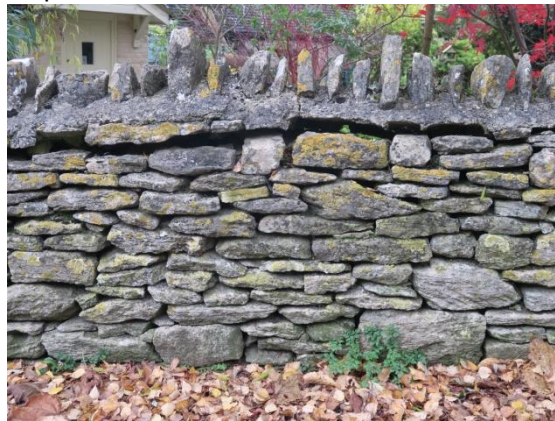
Coping stones set in concrete do not move when the wall does, causing weakness
