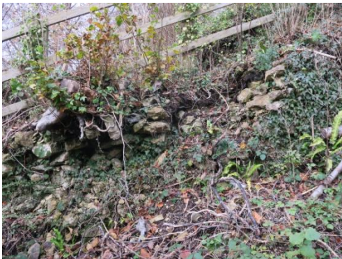
An "ex-wall", due to a weed tree, ivy and lack of timely maintenance
