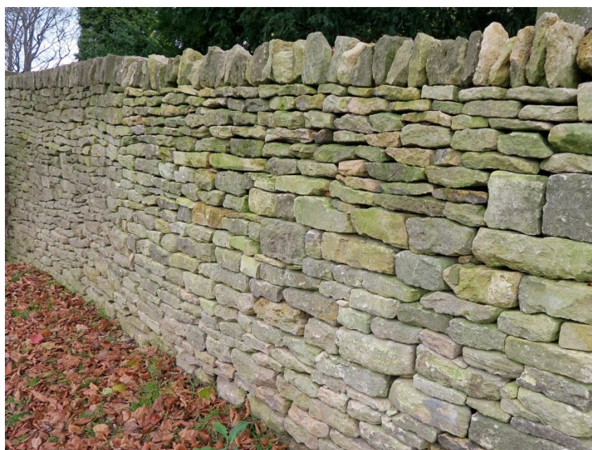
Recently restored wall with mix of stones and vertical toppers
