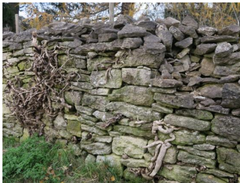
Dead ivy - but too late as wall needs rebuilding
