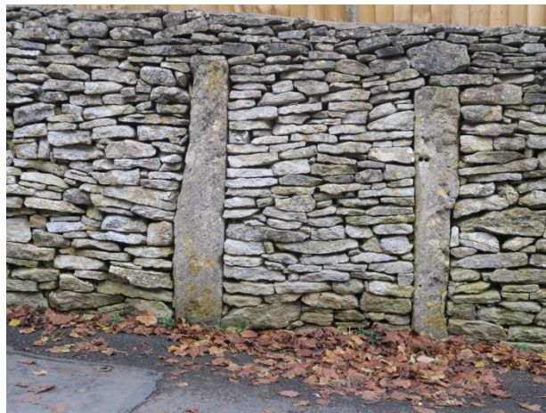
Gate posts - even if no longer used.
