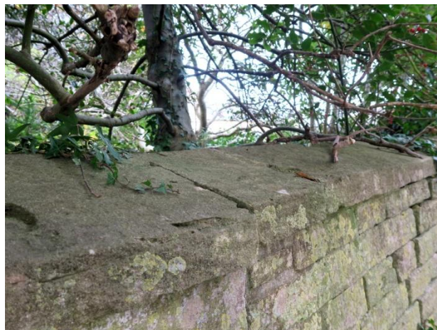
Unusual ridged coping stone near Chalford Primary School
